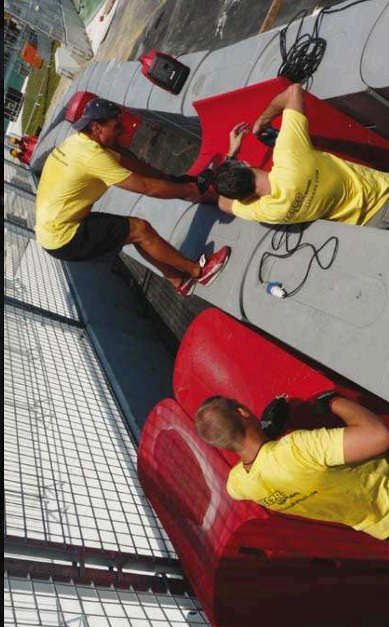
Tecpro's barriers being installed (left), and before and after post-crash intervention (top and above)
